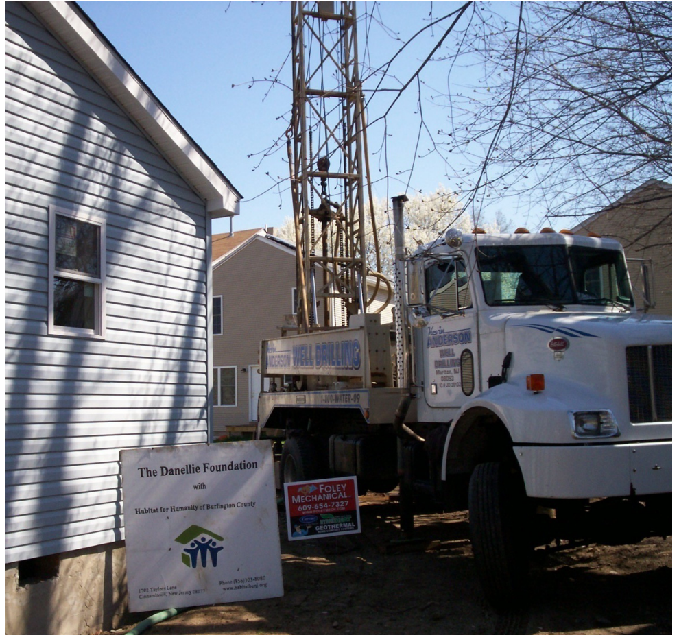
Drilling in Beverly for the installation of geothermal heating system.
